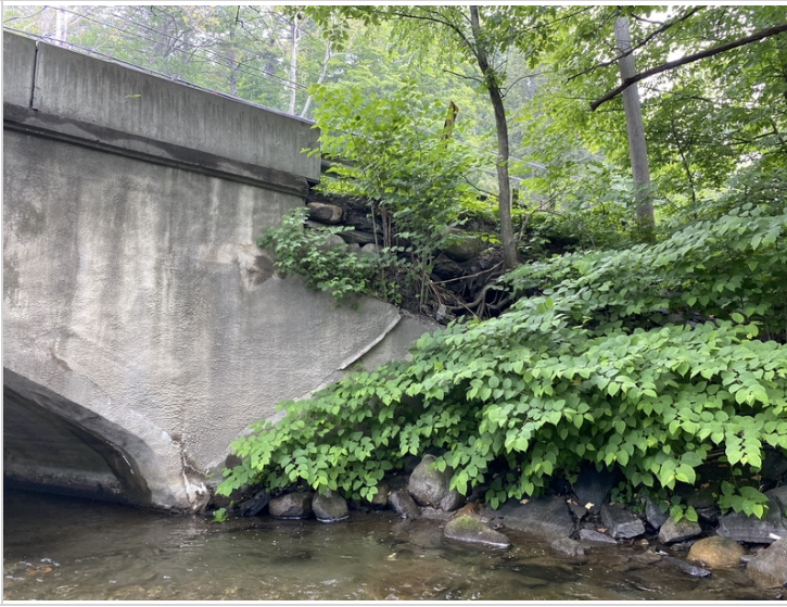
Downstream Eastern Retaining Wall
