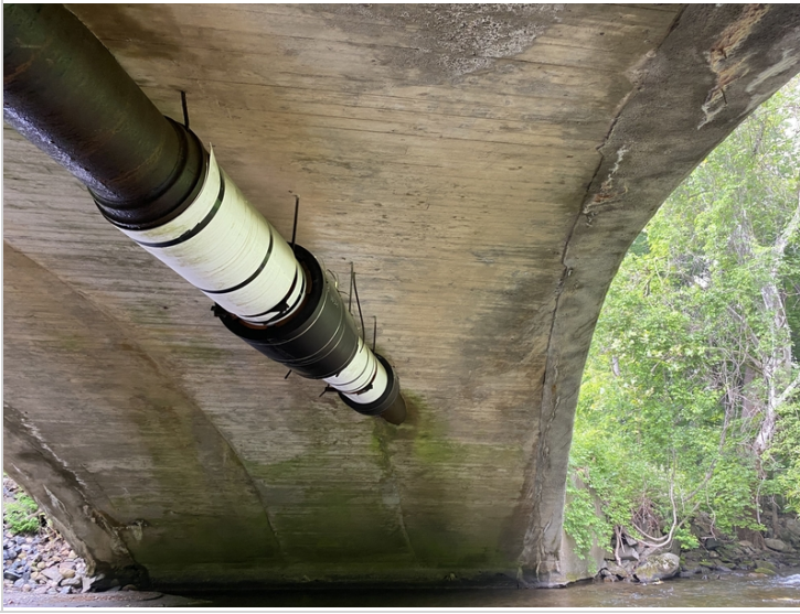
Arch towards West End Upstream
