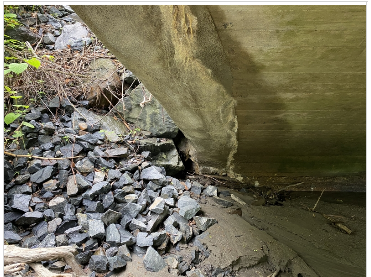
Upstream East End of Arch
