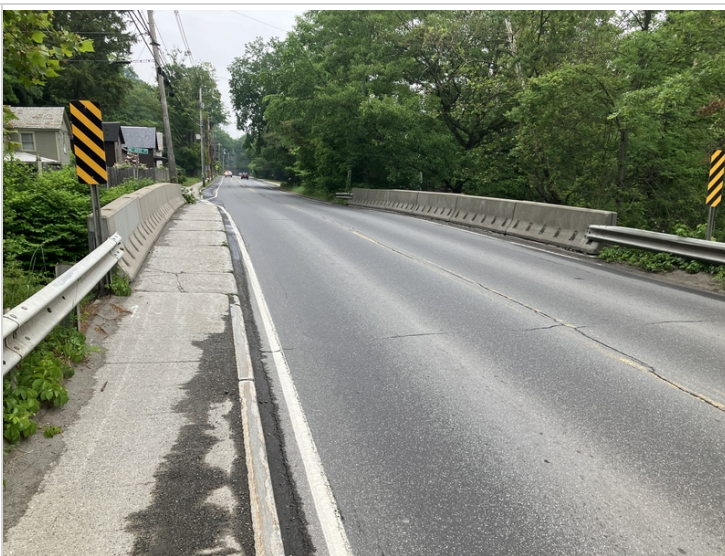
Approach from Abutment 1
