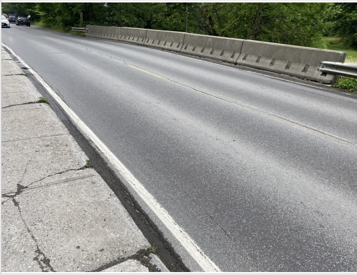
Wearing Surface over Structure
