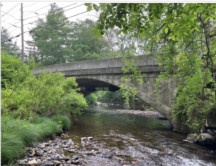
Upstream Bridge Elevation
