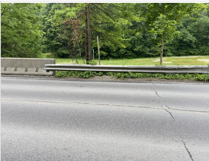
Southwest Transition Rail
