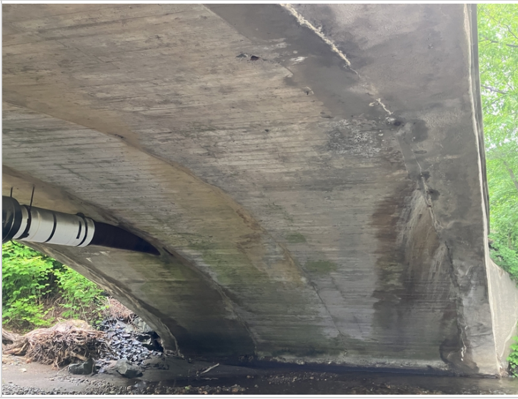
Abutment 2 side of arch
