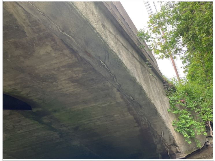
Upstream edge of arch at Abutment 1
